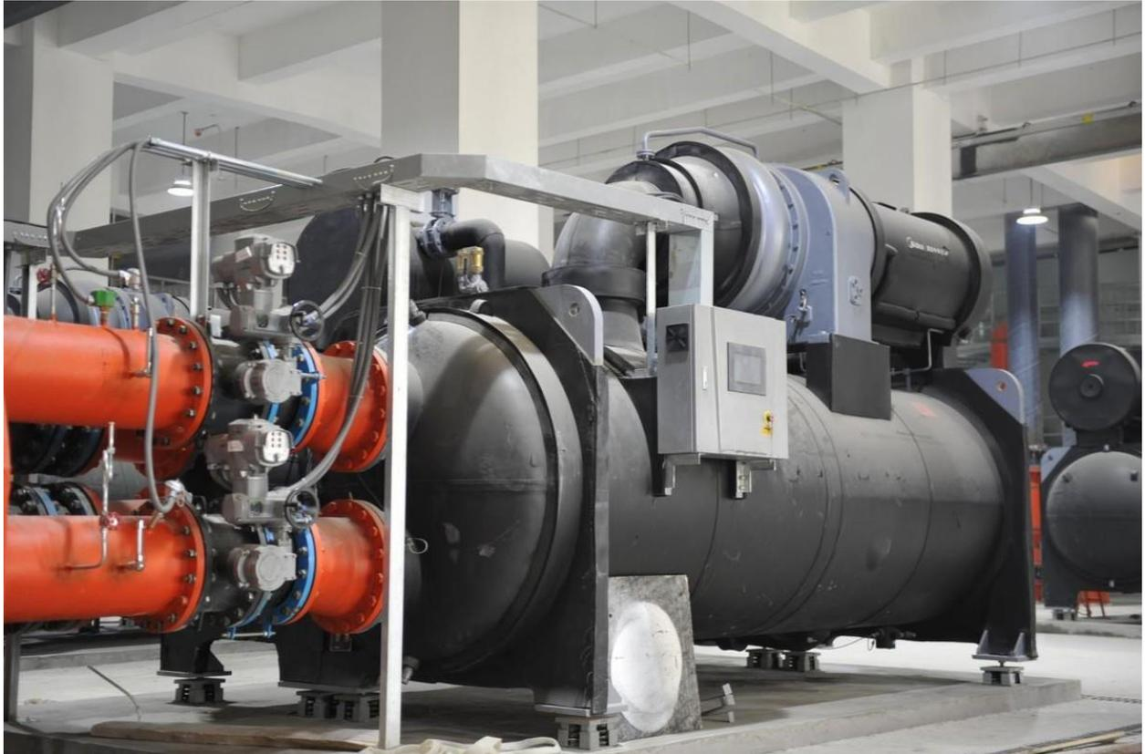
GSHP is an energy-efficient and environment-friendly air conditioning system that uses shallow geothermal energy for heating and cooling buildings. It uses the earth as a heat source in the winter and a heat sink in the summer.
